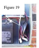
This completes all cable connections and cable routing into the control box.
