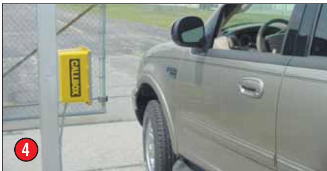
Security code is received by the OutPost wireless callbox. The built-in GateGuard feature activates the "attached" gate controller. The gate opens allowing approved visitors to enter facility.
